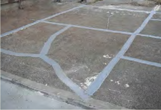
Repair of flat roof to stop leaks.
