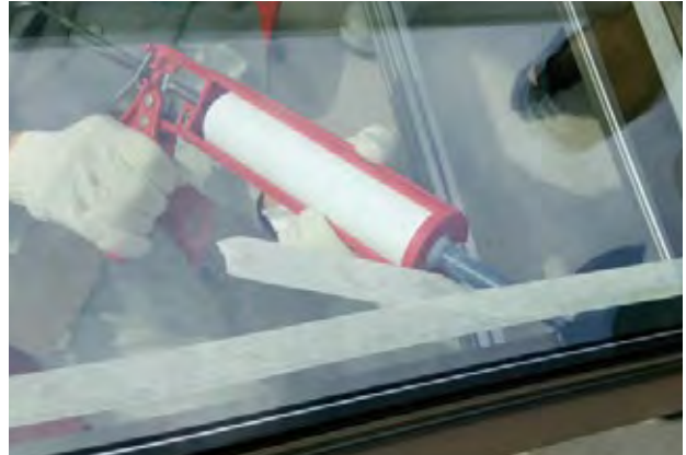
The joint must be filled with no gaps or air.
