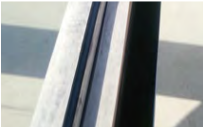
Remove masking tapes immediately after tooling.
