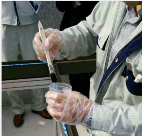
The primer should be transferred to a smaller container. The amount should not exceed what can be applied within 10 minutes.
