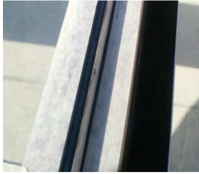
Remove masking tapes immediately after tooling.
