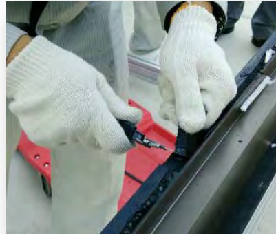
Check the sealant adhesiveness for both glass and substrates.
