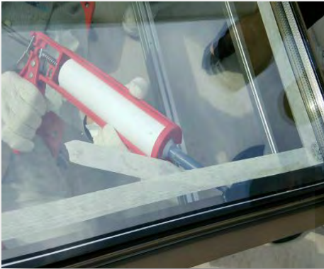
The joint must be filled with no gap and air.
